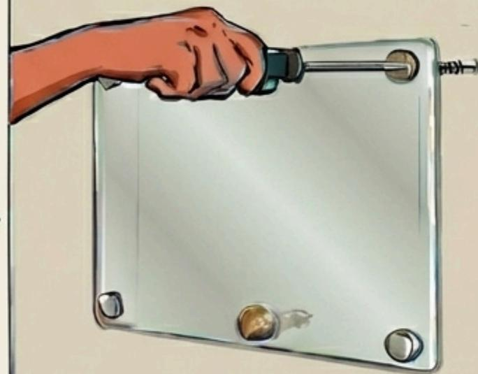
Screw in each cap base. (Hand tighten the last bit) and then screw on each mount cap.
