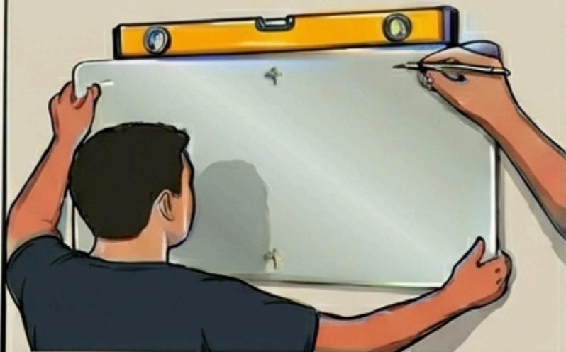
Position panel with spirit level. Mark center points of each mounting hole with a pencil.
